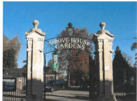
Gates following restoration
