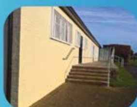
Refurb of Kingsbury Pavilion changing rooms
