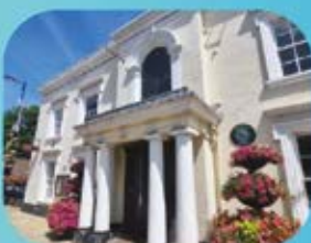
Preservation of Grove House & launching as a wedding venue
