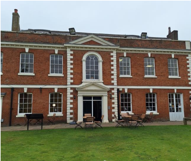
PRIORY HOUSE CENTRAL ARCH WINDOW
